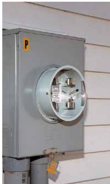
Surge suppressor mounted near the electrical source.
