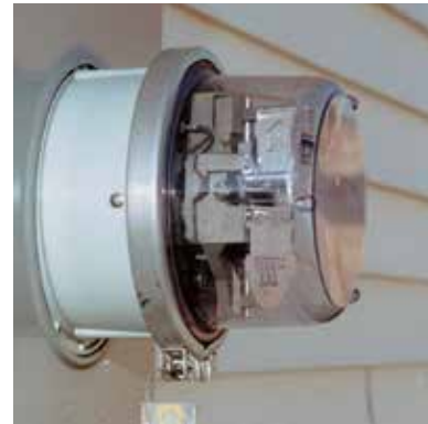
Surge suppressor mounted behind the meter.
