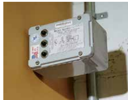
Surge protector mounted at the electrical panel.
